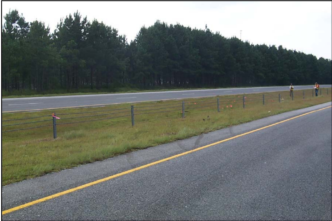
Figure 1: Three-strand cable guardrail.
